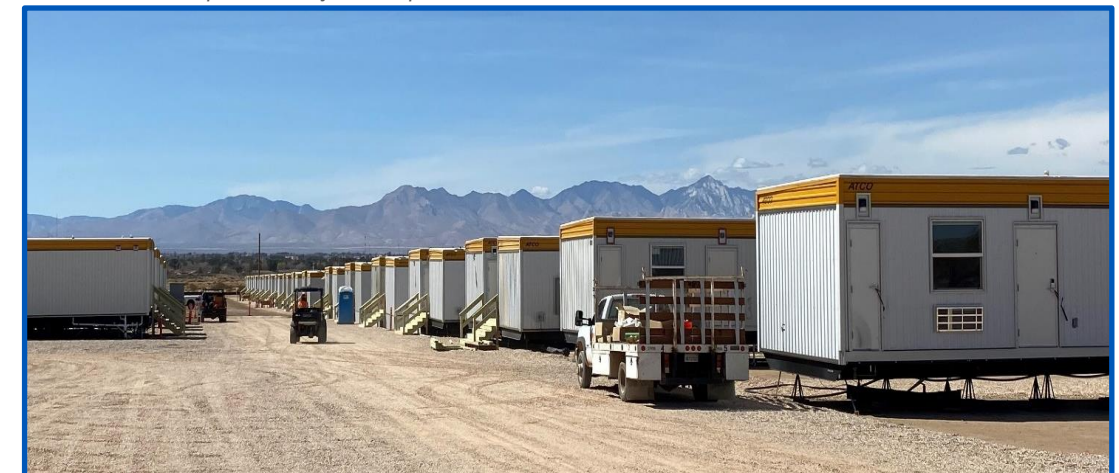
China Lake Military Rebuild, Southern California, US
