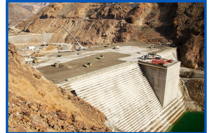
ROLLER COMPACTED CONCRETE
