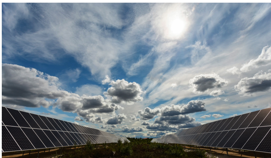
Old Crow Solar Project - Old Crow, Yukon
