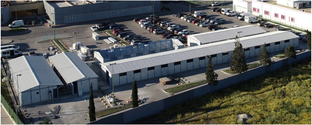
Modular Health Care Facility, Tijuana, MX
