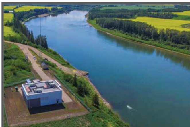
INDUSTRIAL WATER SERVICES CANADA 85,200 m 3 /day
