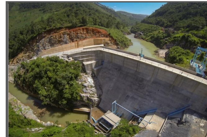
ELECTRICITY GENERATION MEXICO 41 MW
