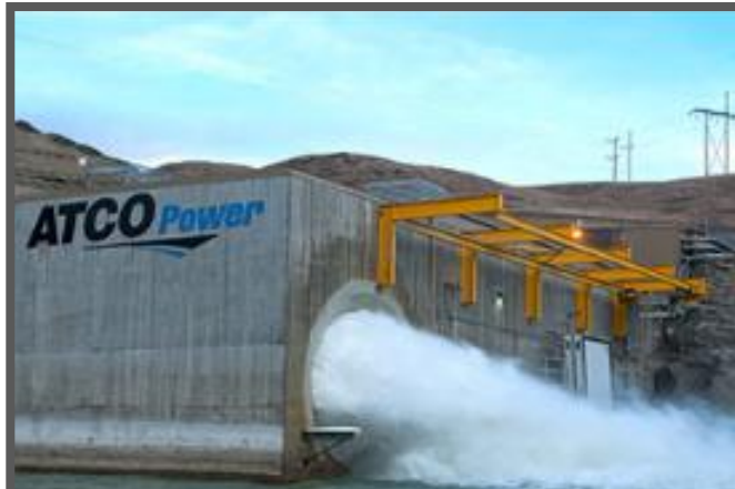
ELECTRICITY GENERATION CANADA 24 MW
