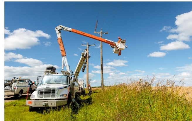
ELECTRICITY DISTRIBUTION $2.6B Rate Base
