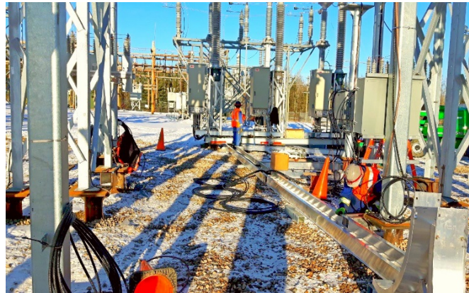
ELECTRICITY TRANSMISSION $5.1B Rate Base
