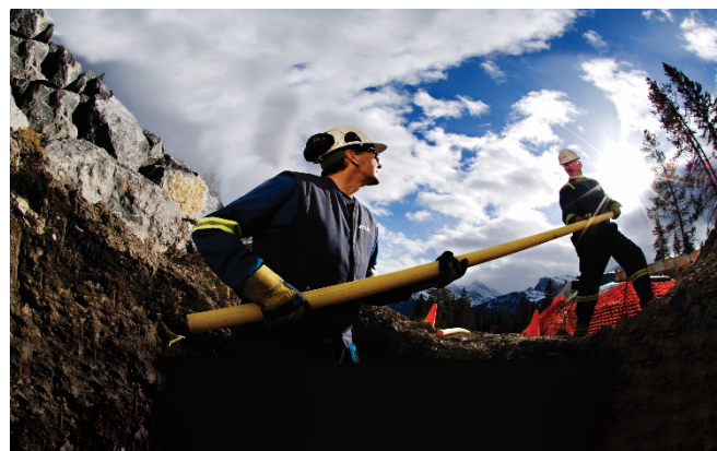
NATURAL GAS DISTRIBUTION $2.9B Rate Base
