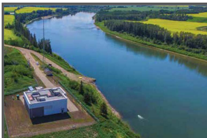
INDUSTRIAL WATER SERVICES CANADA 85,200 m 3 /day
