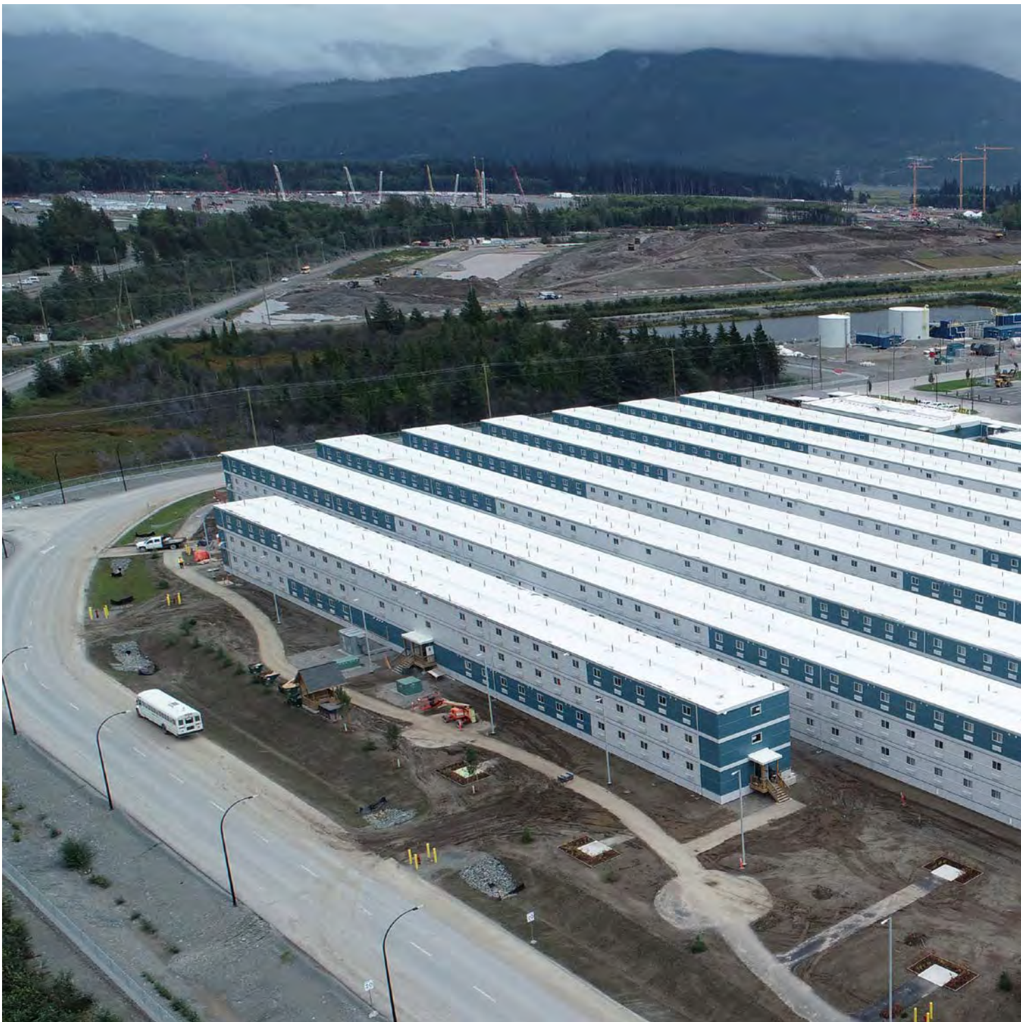
Through our joint ventures with Bird Construction Inc. and the Haisla Nation, we completed the first phase of the LNG Canada Cedar Valley Lodge in 2020, which will ultimately become one of the largest worker accommodation centres in Canada.
