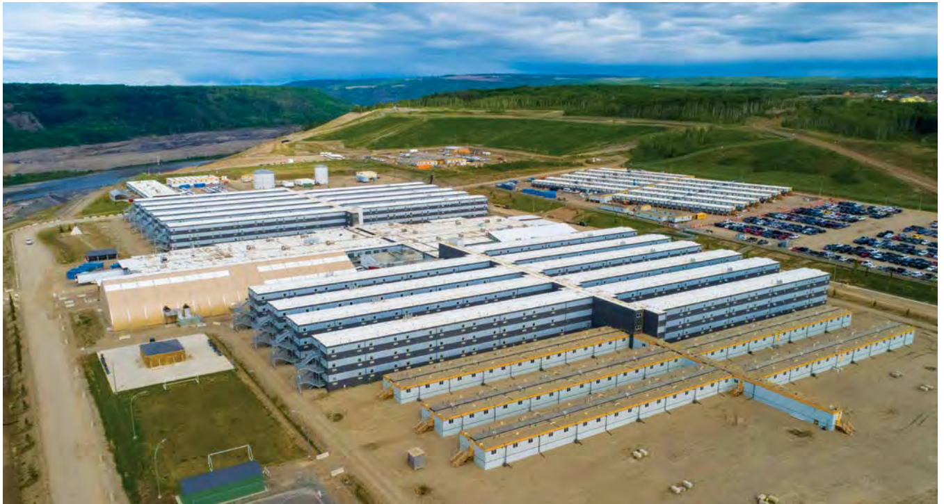
ATCO provided the workforce housing and camp services at Two Rivers Lodge for construction crews building BC Hydro's massive Site C clean energy project.
