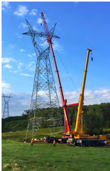
Alberta PowerLine's Fort McMurray West 500-kV transmission project.
