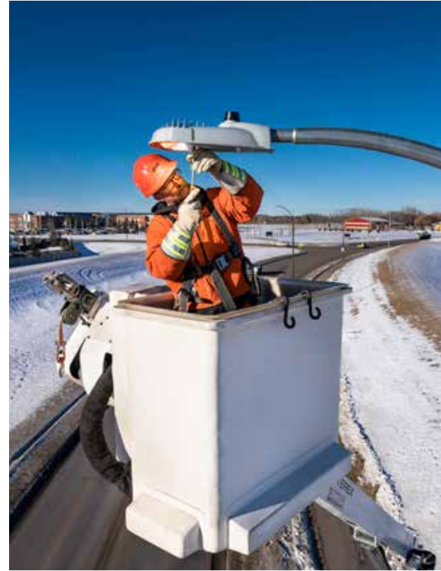
In Lloydminster, we converted outdated street lights to LED bulbs and installed intelligent street lighting sensors. The combined technologies reduce costs, maintenance
